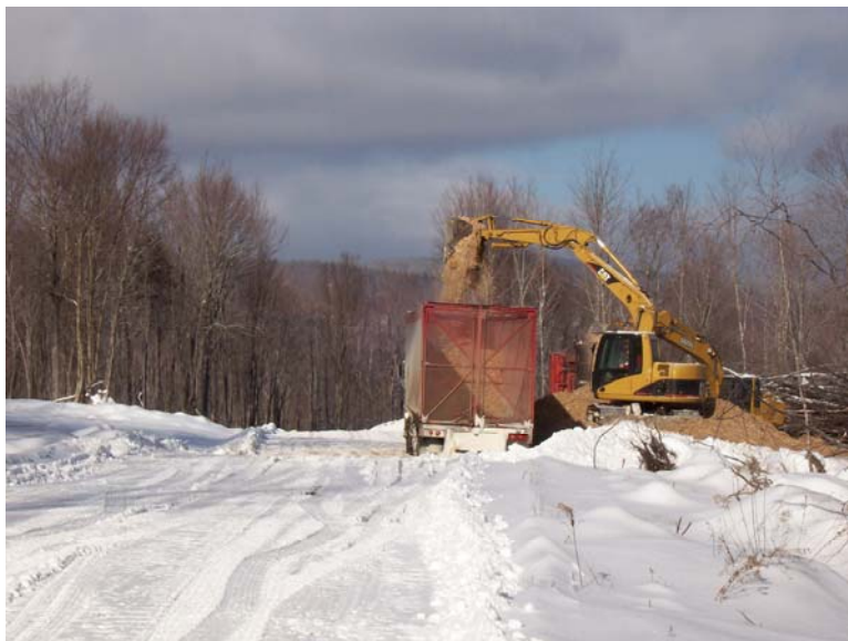
Figure 6: Excavator loading a chip-truck
