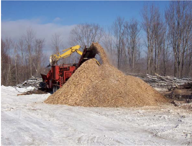
Figure 3: Excavator feeding brush into the grinder
